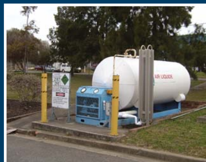
The pH of caustic waste is reduced by injection of liquid carbon dioxide.
